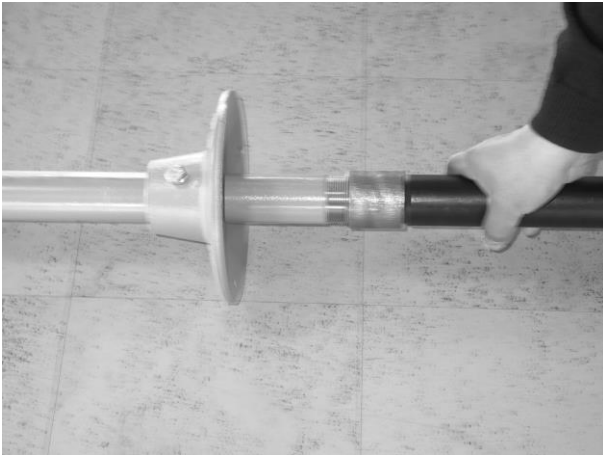
Figure 9: Fastening of the main pipe
